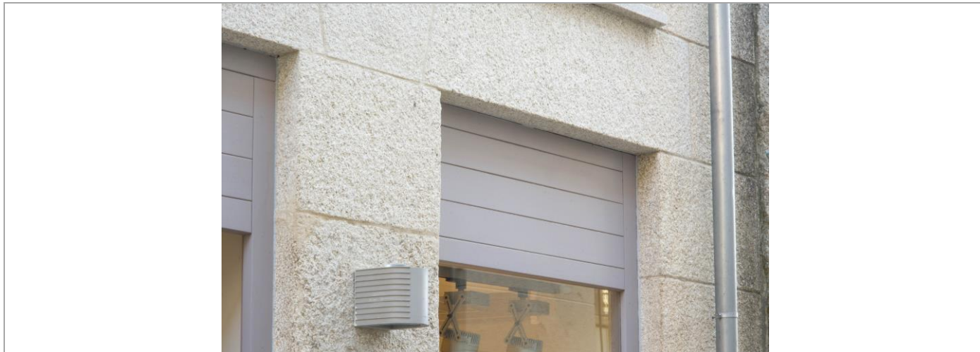
Elemento FACHADA / LUMINARIA / C Cor Elemento: S 2005-R50B; S 2502-B; S 4000-N; S 4005-R50B; S 3010-Y20R
